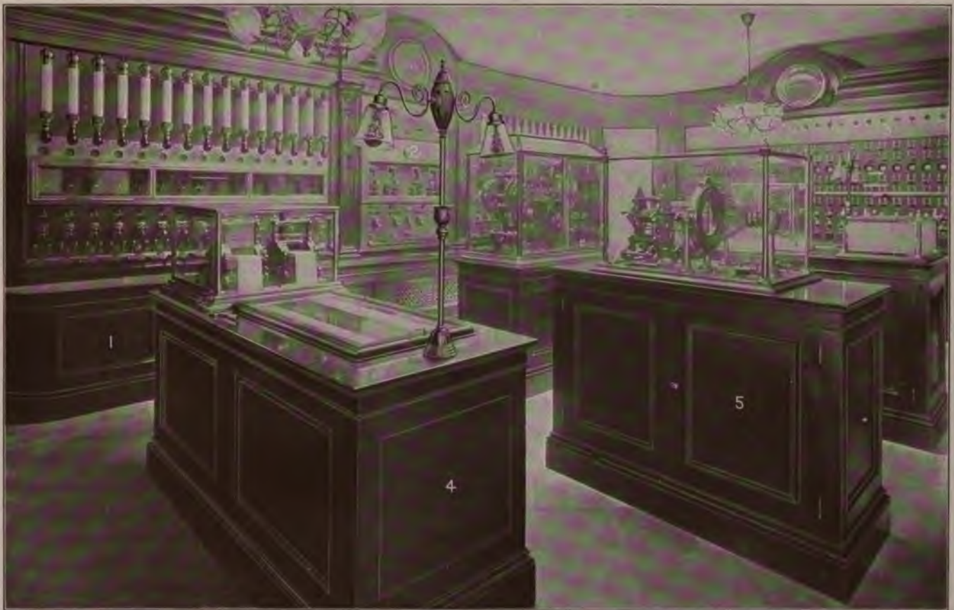
1, Relay switchboard; 2, joker board; 3, working switchboard; 4, multiple pen register; 5, automatic line tester.
